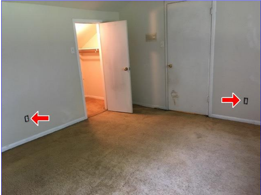
B. Item 24(Picture) Two cover plates missing for electrical outlet receptacles in upstairs right bedroom.
