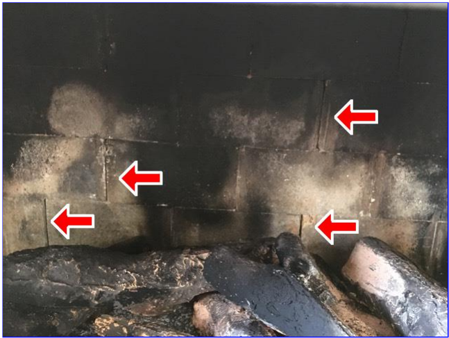
J. Item 3(Picture) Firebricks in fireplace need to be pointed up again. Missing mortar between the fire bricks.
