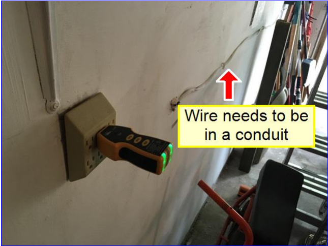
B. Item 10(Picture) Electrical outlet receptacles in the garage not wired for GFCI. In addition wiring along right wall needs to be in a conduit.
