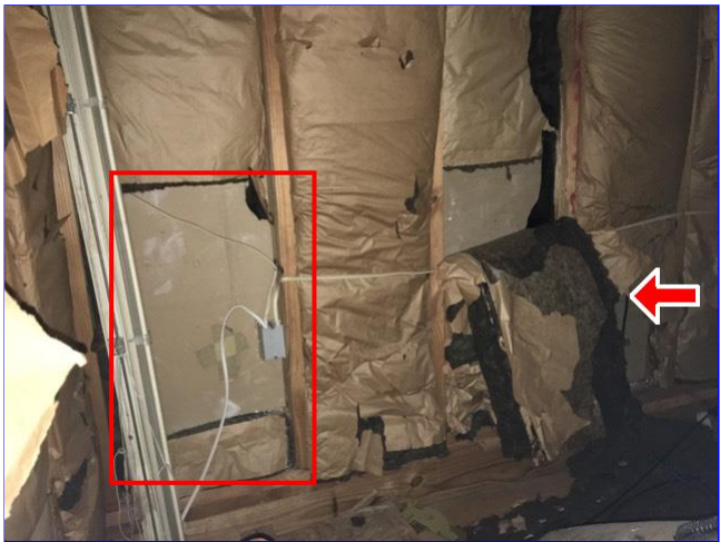
E. Item 16(Picture) Hot walls missing insulation at upstairs right bedroom attic area.
