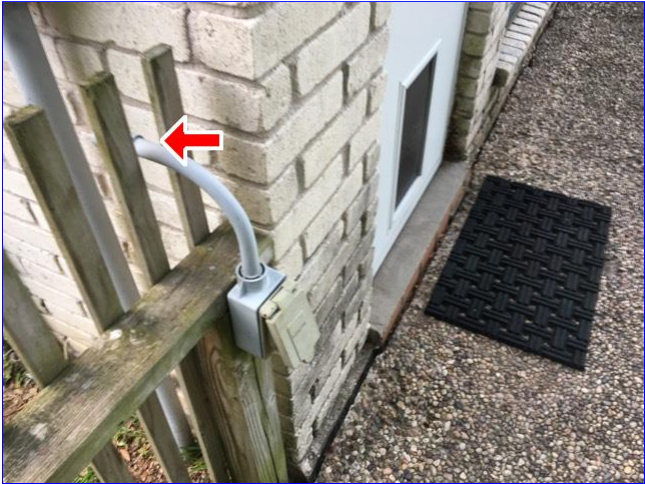
B. Item 1(Picture) Exterior switch at rear right of home not wired to anything
