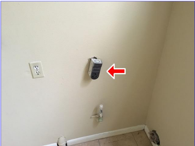
B. Item 11(Picture) Dryer plug needs to be secured to the wall in utility room.
