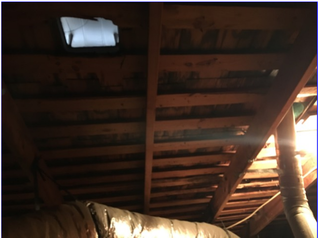
C. Item 16(Picture) NOTE: Original wood shingles still installed underneath architectural shingles on exterior of home.
