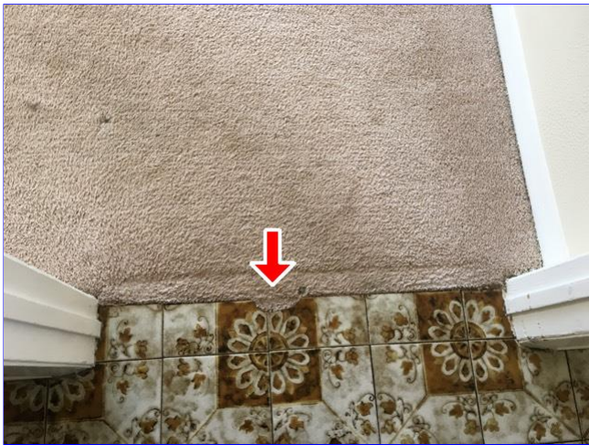
F. Item 9(Picture) Crack at tile between dining room and hallway.
