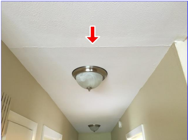
F. Item 4(Picture) Crack in ceiling of hallway on right side of home.
