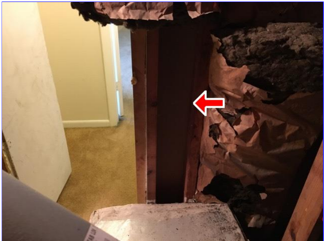
E. Item 15(Picture) Insulation missing at hot wall at left attic.
