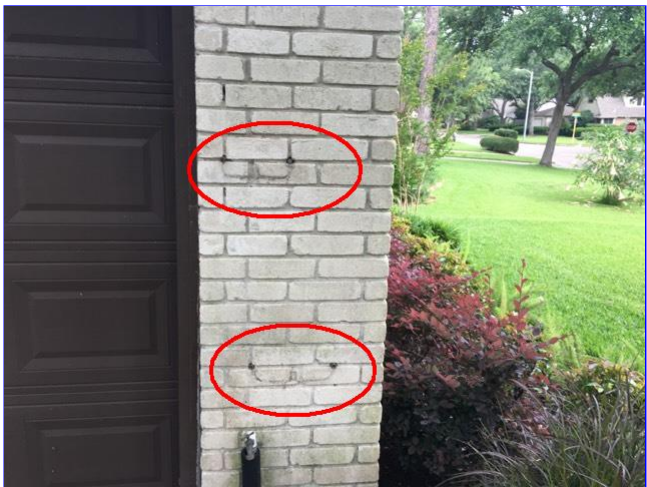
E. Item 8(Picture) Holes drilled into brick in multiple areas around the of home.
