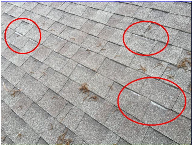
C. Item 4(Picture) Shingles delaminating at left slope above garage.
