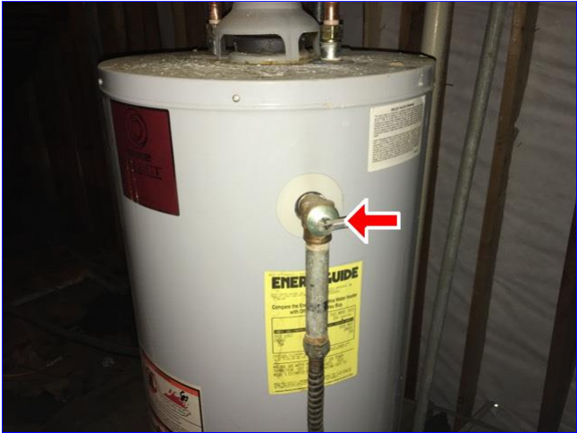
C. Item 1(Picture) T/P valve for water heater leaking.
