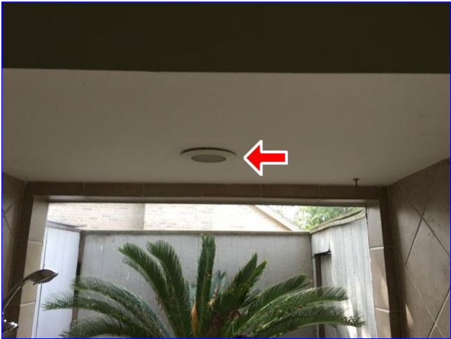
B. Item 20(Picture) Appears recess bulb at master shower area burnt out.
