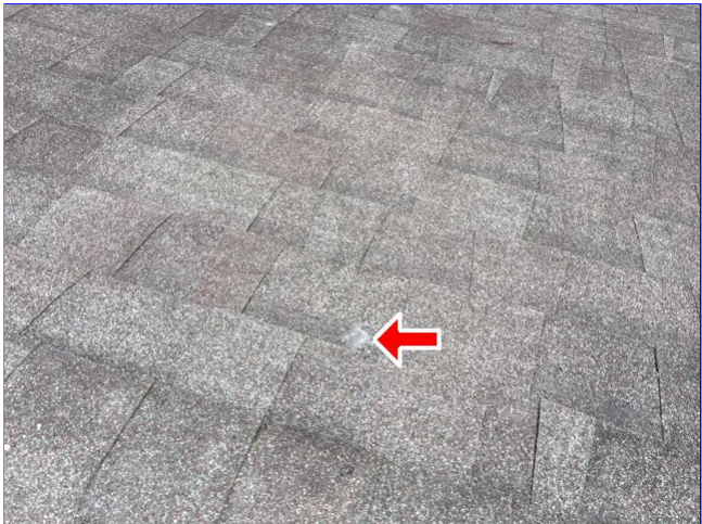
C. Item 6(Picture) Impact damage at right slope of home.
