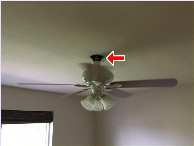
B. Item 23(Picture) Estcushion missing for ceiling fan in upstairs right bedroom.
