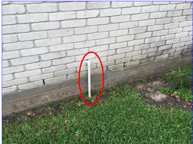
A. Item 1(Picture) Conduit for irrigation system needs to be painted.
