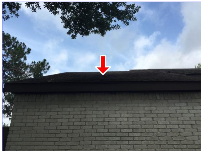
D. Item 1(Picture) Roof deflecting, beginning to sag at the front left slope of home.
