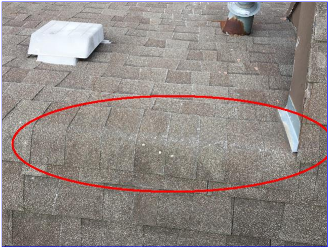
C. Item 12(Picture) Ridge shingles delaminating at middle ridge at home
