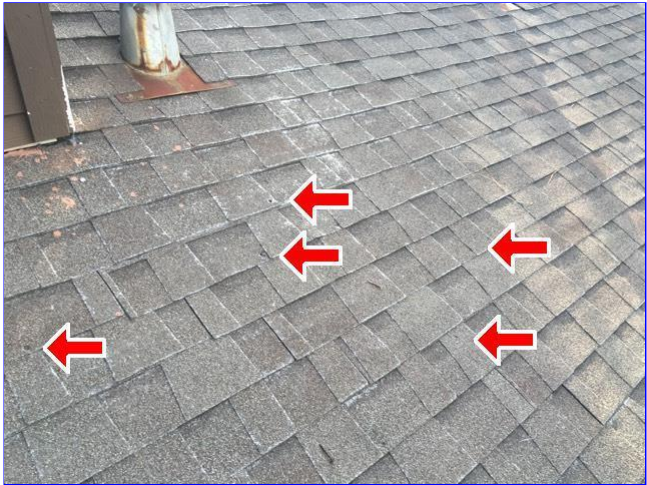
C. Item 21(Picture) Multiple nails hammered through shingles and rear left slope of home.
