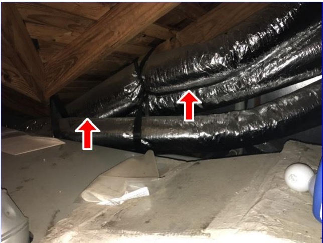
C. Item 1(Picture) Ducks touching each other at right HVAC unit.
