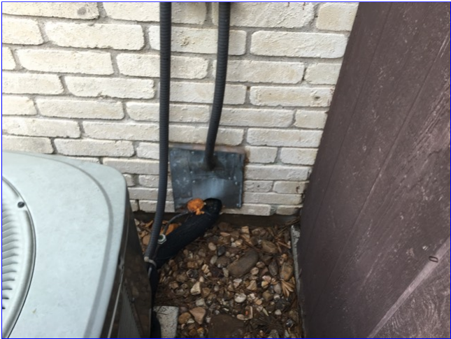
B. Item 2(Picture) Copper box for A/C compressor on the left side of home needs to be painted
