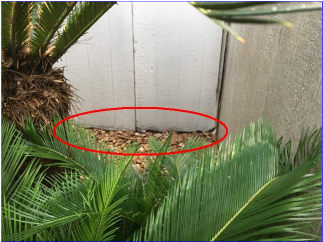
E. Item 4(Picture) Rot noted around partition walls on left side of home.
