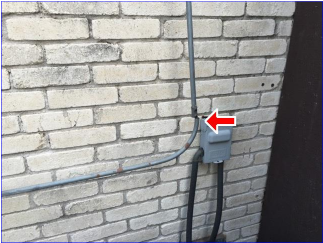
B. Item 2(Picture) Electrical conduit at left side of home needs to be secured to wall. In addition conduit piping needs to be reconnected at coupling.
