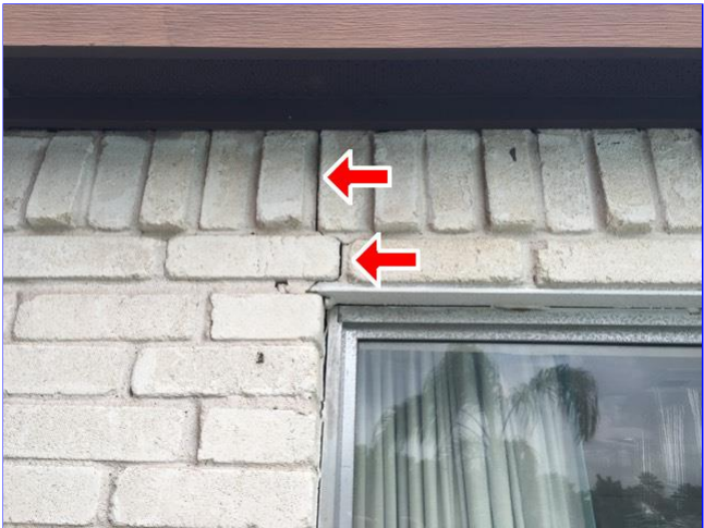
E. Item 5(Picture) Cracks in brick at rear of home.
