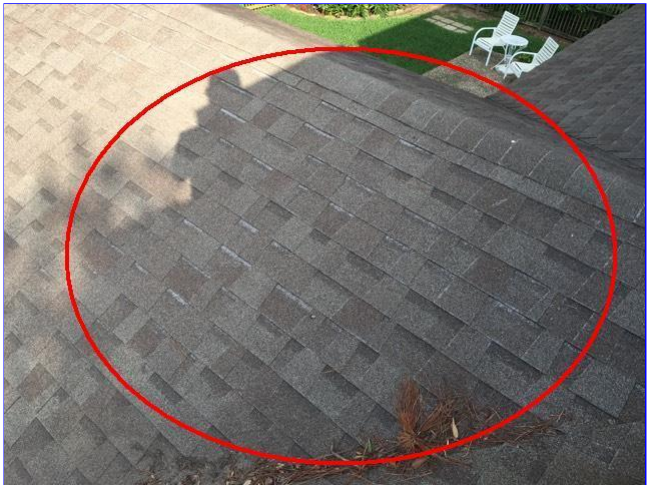
C. Item 18(Picture) Shingles delaminating at rear left slope of home.
