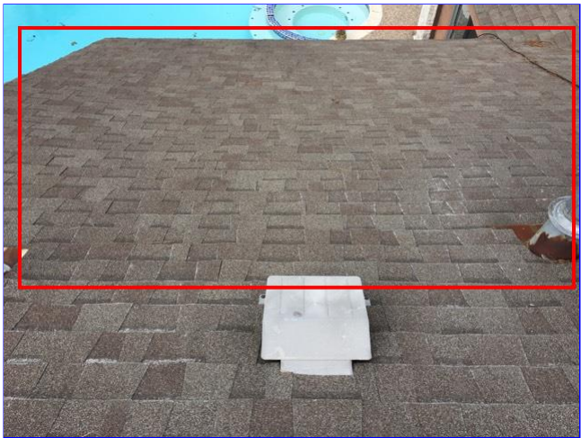
C. Item 13(Picture) Rear slope of home shingles delaminating.
