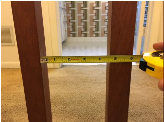
I. Item 1(Picture) Stair parts wider than 4 inches apart.
