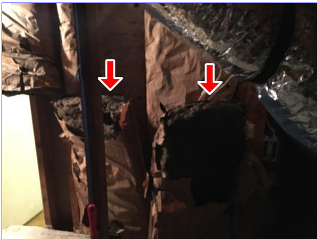
E. Item 14(Picture) Hot wall insulation coming away from wall at left attic.
