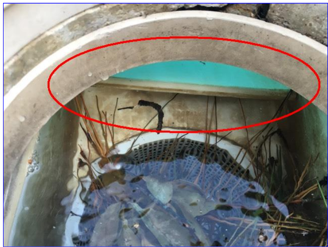
B. Item 2(Picture) Weir wedged between walls of strainer. Also basket needs to be cleaned out
