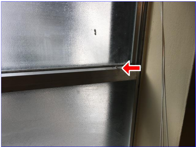
H. Item 4(Picture) Window latch missing at right hall bath. In addition storm window does not open.
