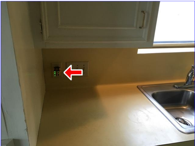
B. Item 7(Picture) Electrical outlet receptacles not wired for GFCI in kitchen. In addition, electrical outlet receptacle has an open ground wire.
