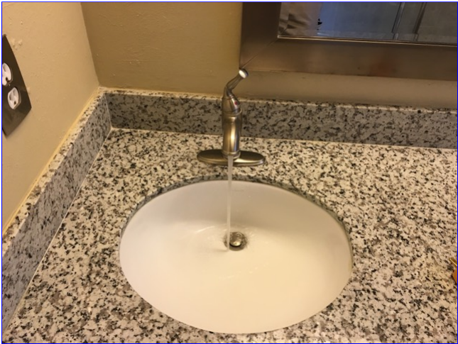
A. Item 4(Picture) Hot and cold reversed at right hall bath faucet.
