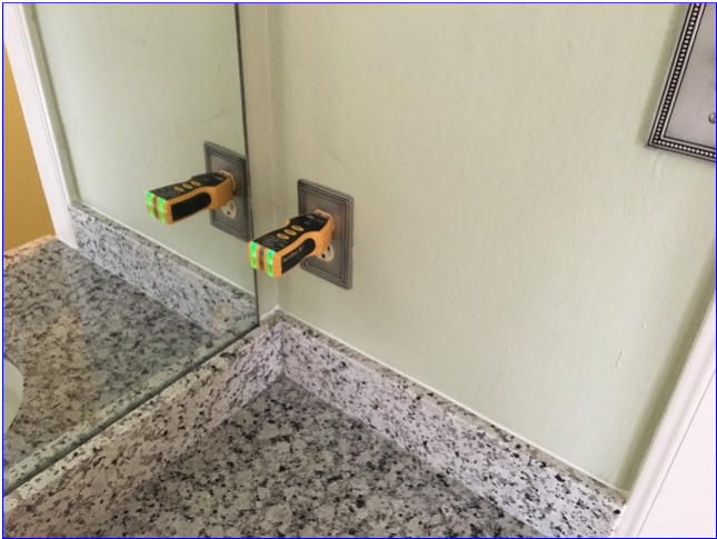
B. Item 17(Picture) Electrical outlet receptacles in master bath not wired for GFCI.
