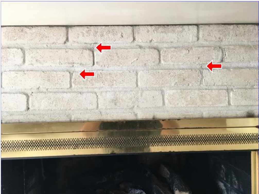
J. Item 5(Picture) Cracks in brick below mantle of fireplace.
