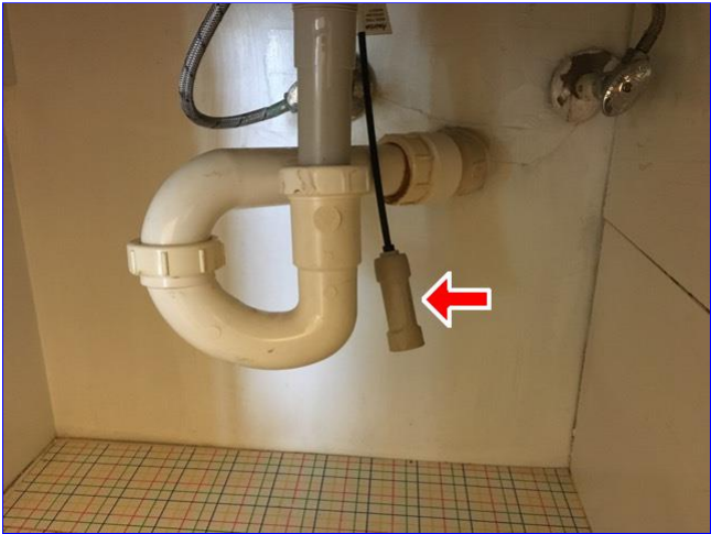
B. Item 2(Picture) Pull handle for stopper not connected at right hall bath.
