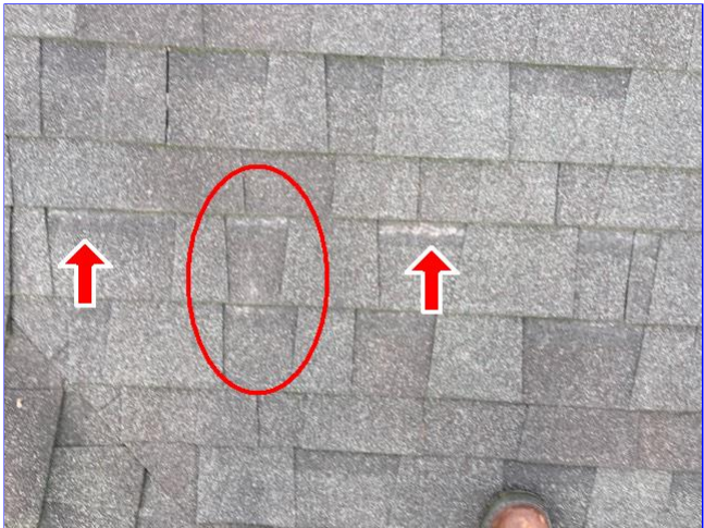
C. Item 8(Picture) Shingles delaminating at the front slope of the home right side.
