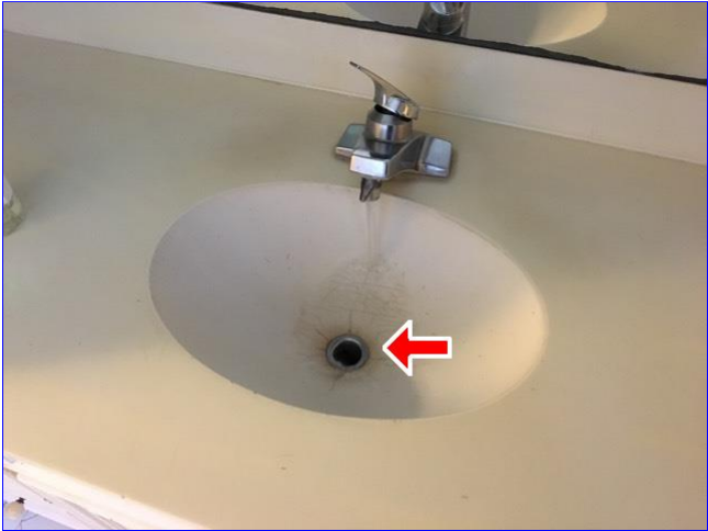
B. Item 6(Picture) Stopper missing in upstairs hall bath.
