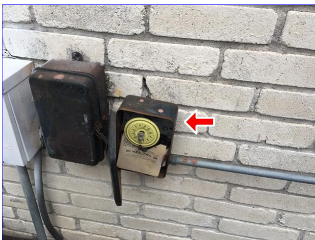
B. Item 7(Picture) Timer box needs to be secured to the wall
