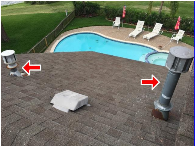
C. Item 11(Picture) Exhaust vents at rear slope of home need to be painted.
