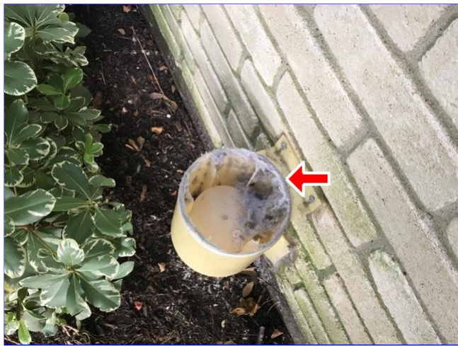
H. Item 1(Picture) Dryer exhaust vent needs to be cleaned out.
