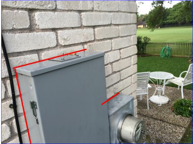
A. Item 3(Picture) Electric service panel box and meter can box should be sealed to the brick. On the right side of the home.
