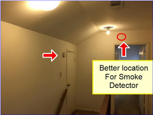
B. Item 29(Picture) Smoke detector in upstairs hallway installed in wrong location. Needs to be within 12 inches of the highest point of the ceiling.
