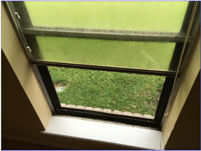
H. Item 2(Picture) Storm window at front right bedroom stuck in the open position.
