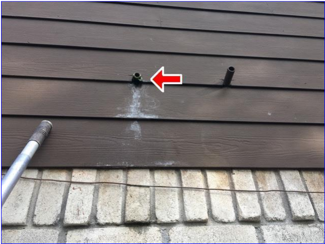
C. Item 2(Picture) T/P valve for water heater leaking.
