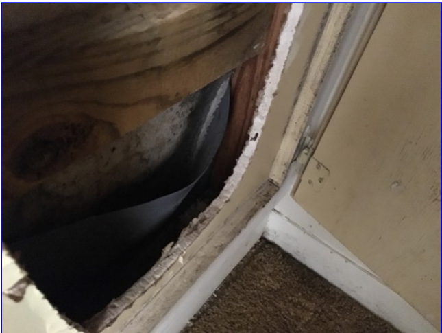
B. Item 5(Picture) Appears to be a water leak behind right hall bath shower.
