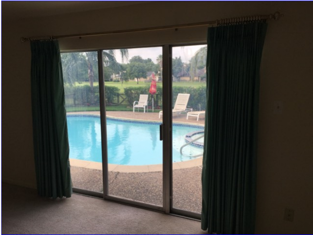
G. Item 9(Picture) Screen missing for sliding glass door at master bedroom.
