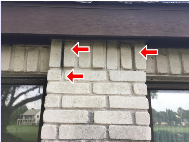
E. Item 1(Picture) Cracks at mortar between the bricks at rear of home.
