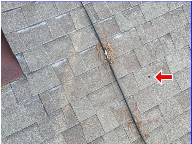
C. Item 19(Picture) Hole goes straight through shingle and decking.
