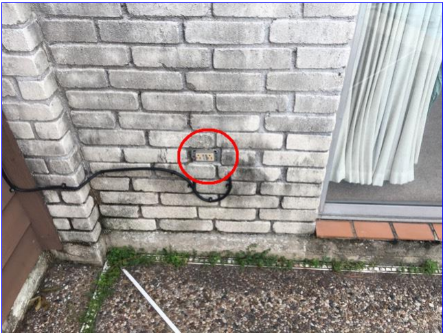
B. Item 4(Picture) Exterior cover plate missing for electrical outlet receptacle at rear of home near pool.
