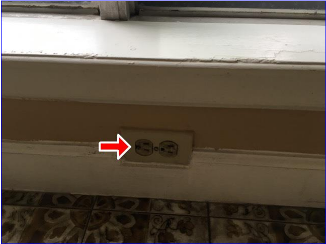
B. Item 8(Picture) Electrical outlet receptacle at breakfast area of kitchen has ground plug broken off in it. In addition, electrical outlet receptacle is loose
