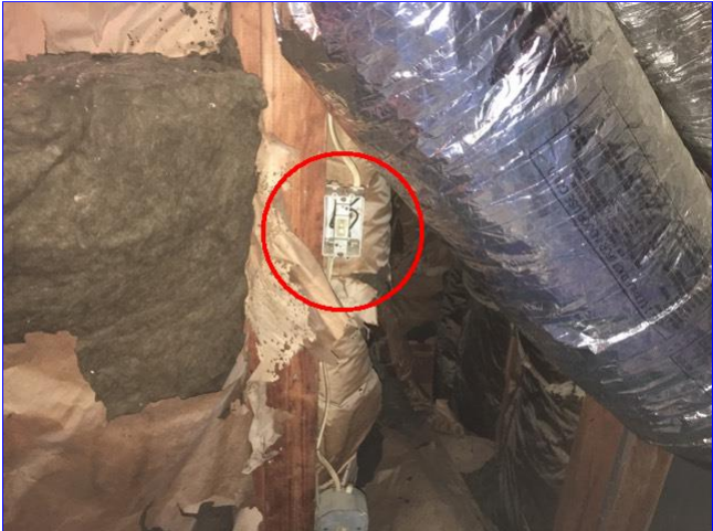
B. Item 22(Picture) Cover plate missing for HVAC cut off switch in attic. Left side attic.
