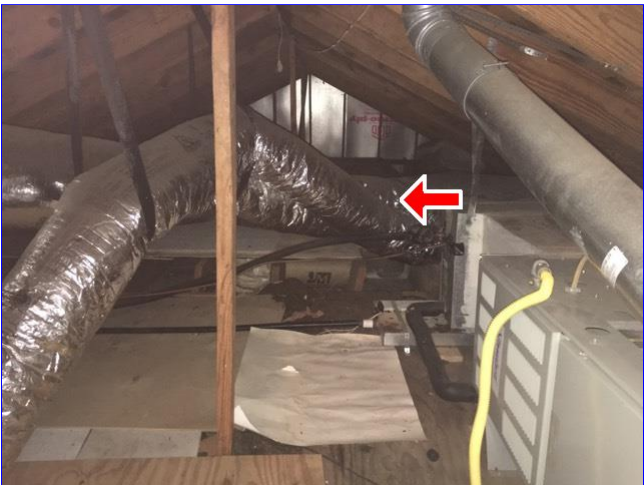
C. Item 2(Picture) Ducts touching each other at right HVAC unit.
