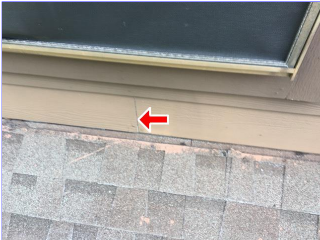
E. Item 12(Picture) Butt joint needs to be caulked at rear slope of home.
