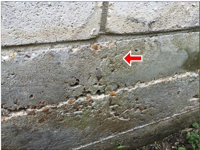
A. Item 4(Picture) Crack in foundation right side of home behind exterior A/C unit.
