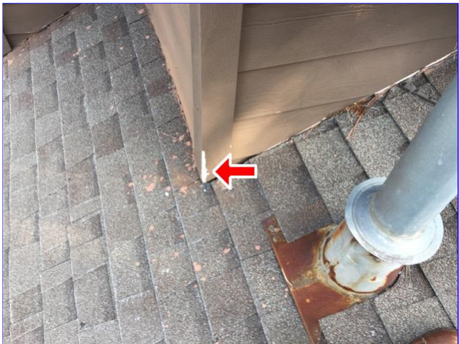
E. Item 10(Picture) Damaged siding at rear left slope of home.
