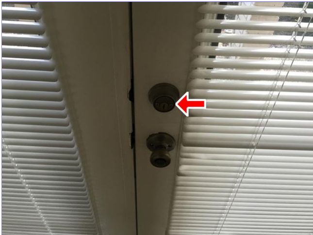
G. Item 3(Picture) NOTE: Double deadbolt at front entry door.
