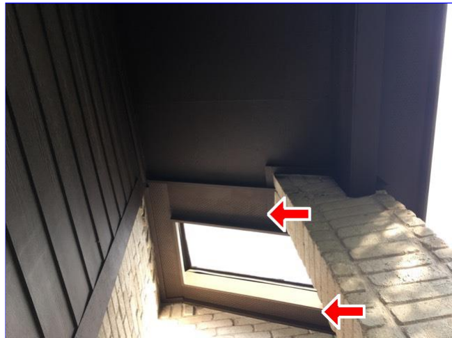
D. Item 2(Picture) Perforated soffit board should not be installed at rakes of a home.
