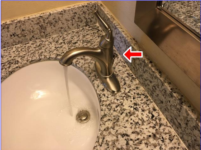
B. Item 1(Picture) Pull handle for stopper at right hall bath sink not working.
