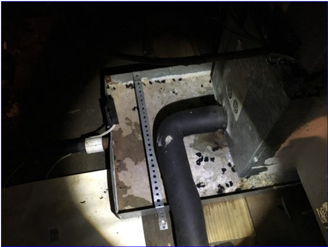
B. Item 5(Picture) Primary drain clogged. Leaking into secondary drain pan.
