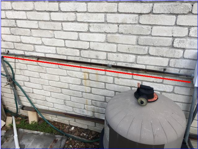
B. Item 3(Picture) Large amount of rust noted at conduit line for pool system. Should be sanded and painted to preserve it
