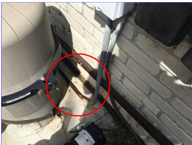
B. Item 8(Picture) Conduit for pool timer rusted through. Needs to be replaced.
