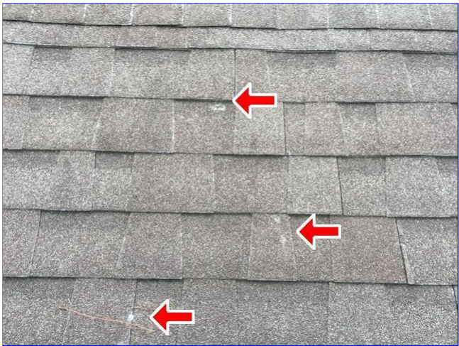
C. Item 23(Picture) Impact damage at rear right slope at home.
