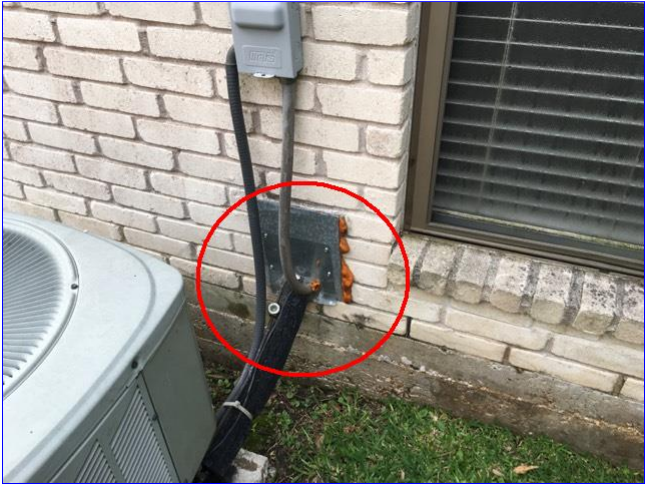
B. Item 1(Picture) Copper box for A/C compressor needs to be painted on right side of home.
