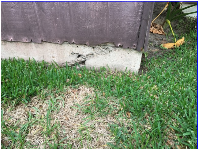
L. Item 1(Picture) Cold joint poor at stem wall surrounding master bath window on left side of home.
