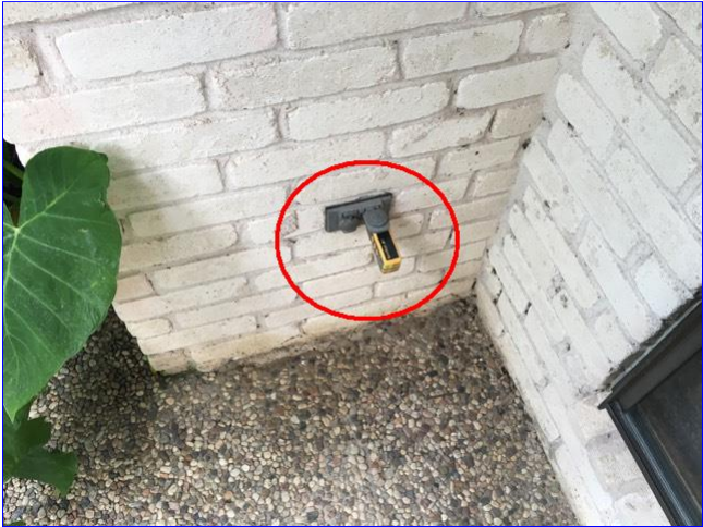
B. Item 6(Picture) Electrical outlet receptacle to the left of front entry door not secured to wall. In addition, GFCI not working.
