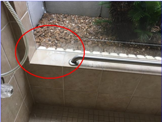
B. Item 3(Picture) Window ledge at master bath not sloped. Holds water when shower is run.
