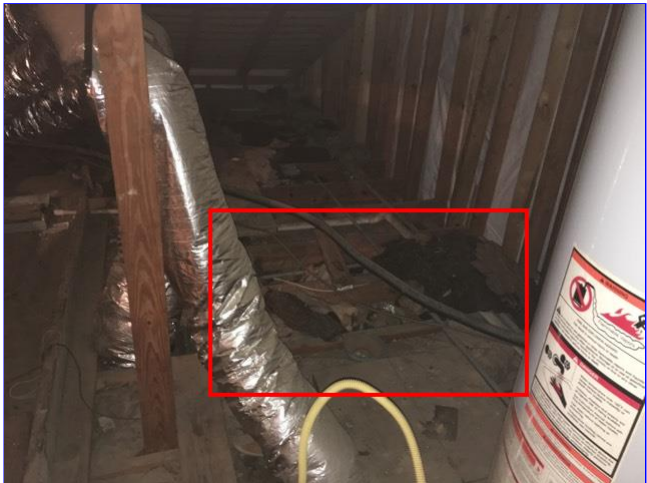
D. Item 3(Picture) Missing insulation above the master bath.
