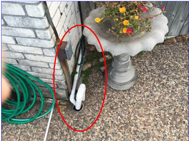
B. Item 5(Picture) It is recommended that PVC piping and a conduit be painted at rear left corner of home.
