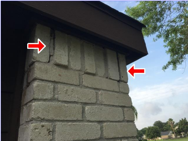
E. Item 2(Picture) Cracks in mortar between brick at rear middle of home.
