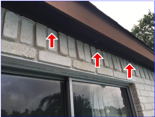
E. Item 6(Picture) Gaps in brick at rear of home need to be pointed up. Above master bed sliding glass door.
