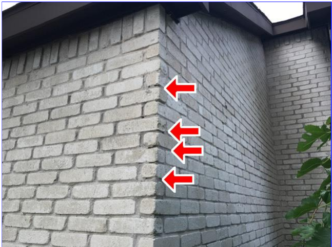
E. Item 9(Picture) Bee holes in brick at front of home.
