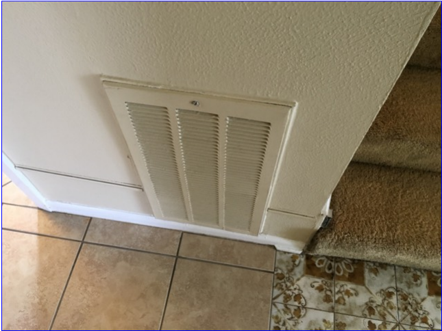
C. Item 3(Picture) Only a 6 degree difference between the return air and supply ducts in living room. Ducts possibly crimped.
