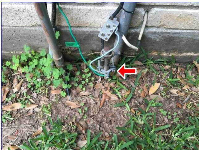
A. Item 1(Picture) Ground rod clamp loose at right side of home near electric service panel box.
