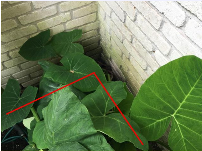
A. Item 2(Picture) Minimum of 4 inches of slab exposure needed at the front of home to the left front entry door.
