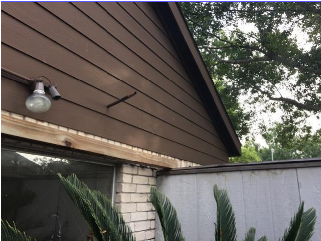
B. Item 6(Picture) Negative slope to secondary drain line for HVAC system on the left side of home. Pipe should be pointed toward the ground.
