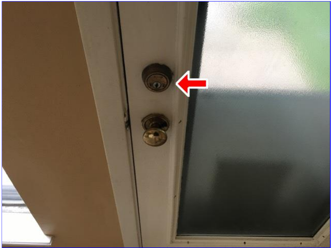
G. Item 5(Picture) NOTE: Double deadbolt at rear exterior door.
