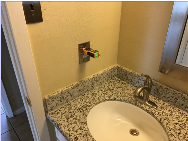
B. Item 12(Picture) Electrical outlet receptacle at right hall bath not wired for GFCI.
