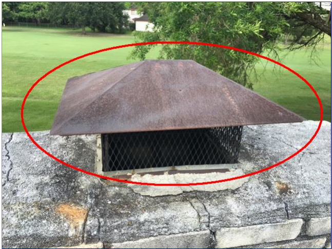
J. Item 1(Picture) Spark arrestor for chimney needs to be painted at rear of home.
