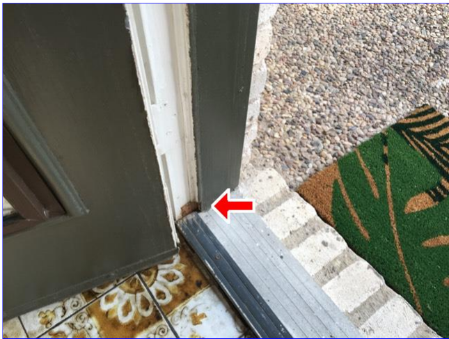
G. Item 2(Picture) Weather stripping missing at bottom right corner of entry french doors.
