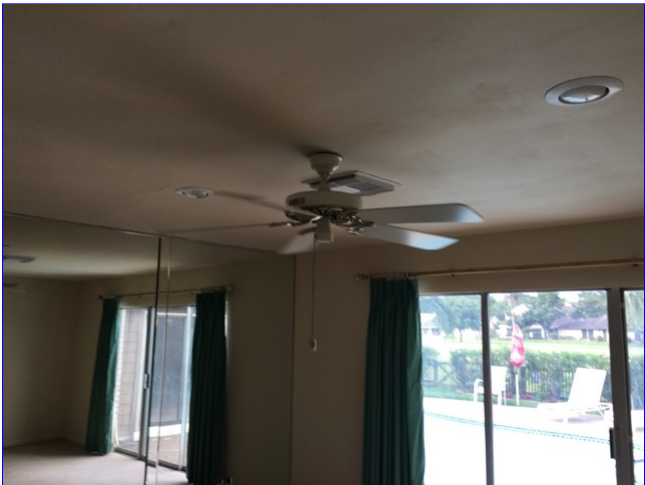
B. Item 21(Picture) NOTE: Ceiling fan in master bed hard wired. Not controlled by switch but by pull chain.
