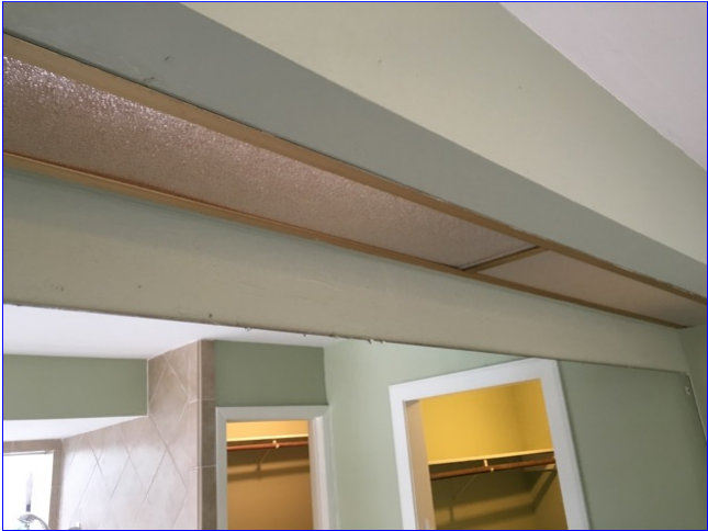
B. Item 19(Picture) Appears fluorescent light ballasts are burnt out at master bath.
