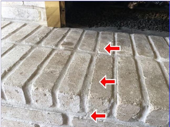
J. Item 6(Picture) Cracks in brick of hearth of fireplace.
