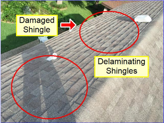
C. Item 15(Picture) Second floor rear slope of home. Shingles are delaminating. Plus damaged shingle first row.
