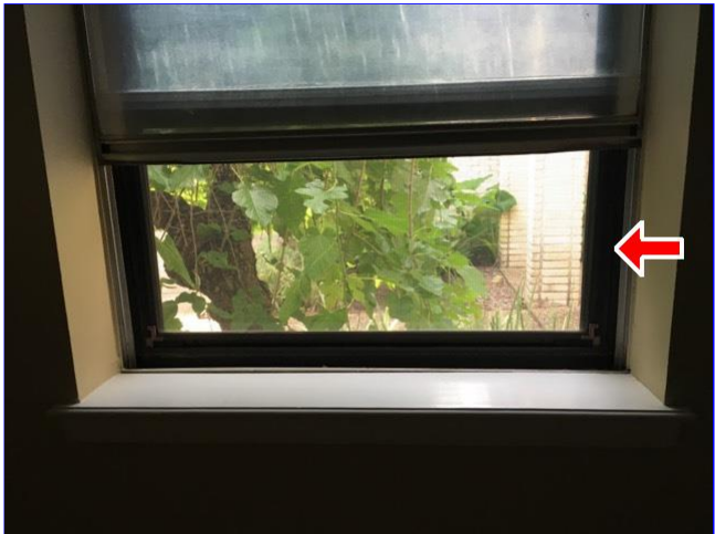
H. Item 3(Picture) Storm window does not open at utility room.
