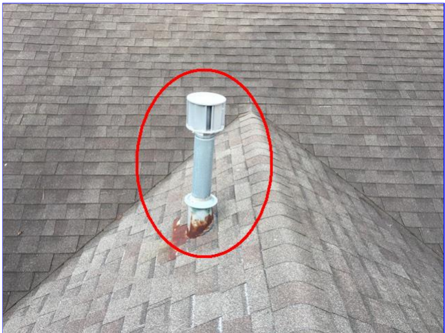
C. Item 7(Picture) Exhaust vent needs to be sanded and painted at front slope of home.
