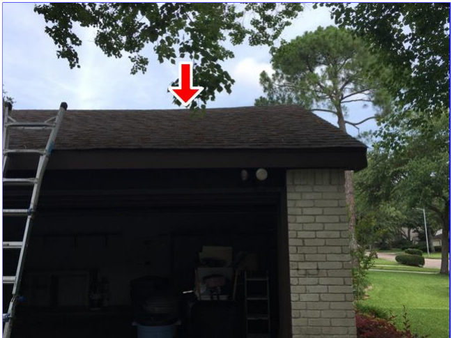
D. Item 5(Picture) Roofline appears to be sagging on right side of garage
