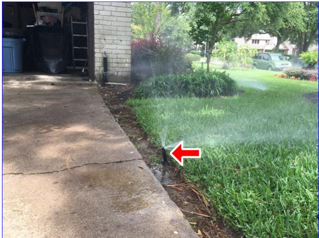
A. Item 3(Picture) Zone two sprinkler head damaged and needs to be replaced.
