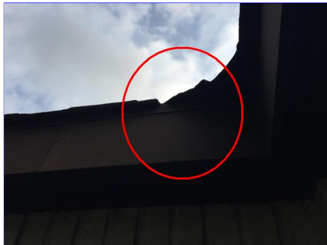
C. Item 2(Picture) Shingles in damaged at rear of home.
