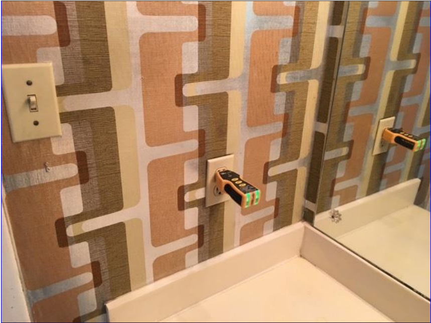
B. Item 26(Picture) Electrical outlet receptacle in upstairs hall bath not wired for GFCI.
