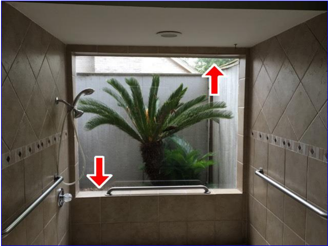
B. Item 4(Picture) Cracks in grout at window sill tile. In addition, appears that upper tiles at window sill are sagging on the right side.
