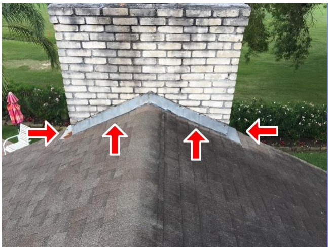
C. Item 14(Picture) Flashing needs to be painted at rear of home.
