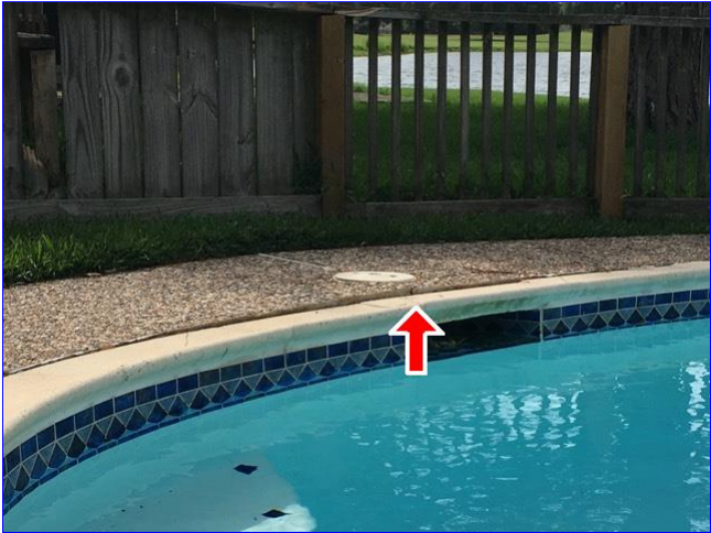
B. Item 9(Picture) Ground heaving around the strainer basket of swimming pool.
