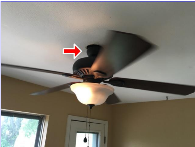
B. Item 27(Picture) Ceiling fan escutcheon needs to be secured to ceiling in breakfast area of kitchen.
