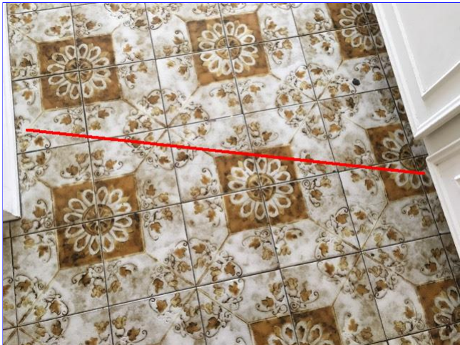
F. Item 8(Picture) Cracked tile floor in between kitchen island and dining area
