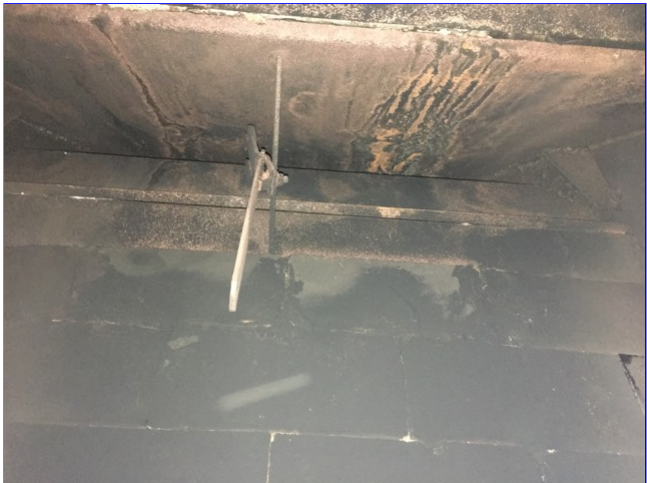
J. Item 4(Picture) Damper difficult to open at fireplace. Could not open.
