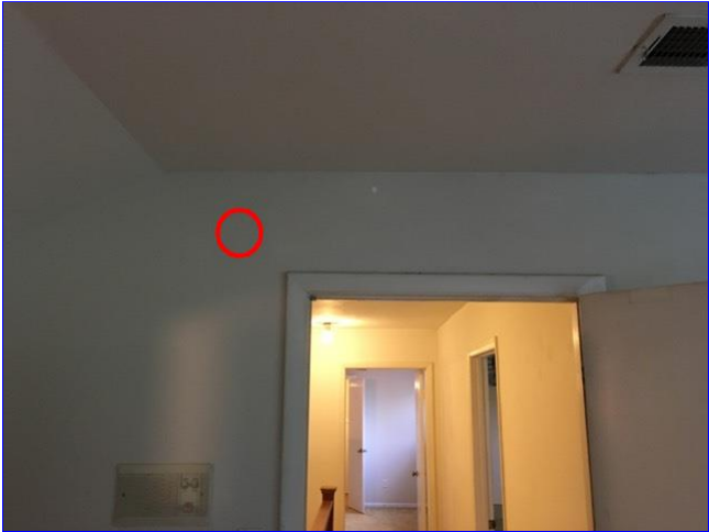
B. Item 28(Picture) Smoke detectors missing at all four bedrooms.
