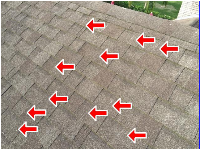
C. Item 9(Picture) Edges of shingles delaminating at front slope of home.
