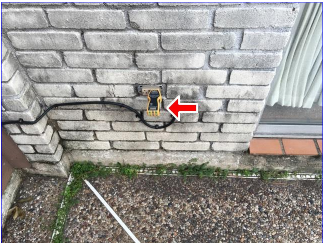
B. Item 5(Picture) GFCI not working at rear electrical outlet receptacle at rear of home.
