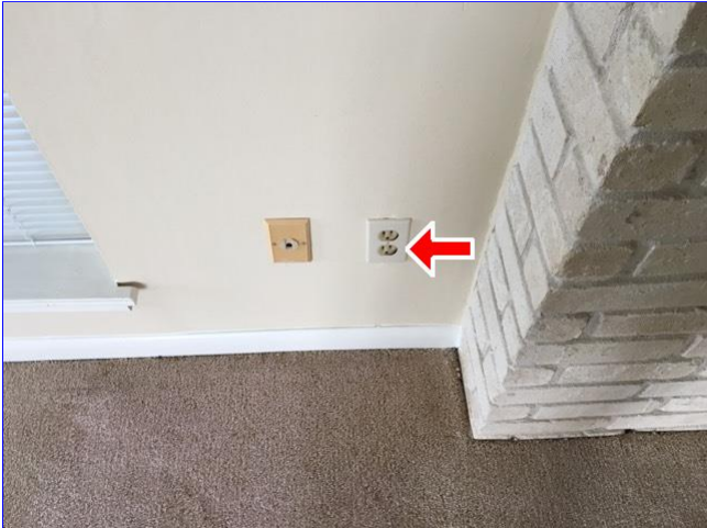
B. Item 13(Picture) No power to electrical outlet receptacle on right wall of family room area.
