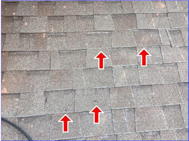
C. Item 20(Picture) Nails hammered through shingles at rear slope of home.
