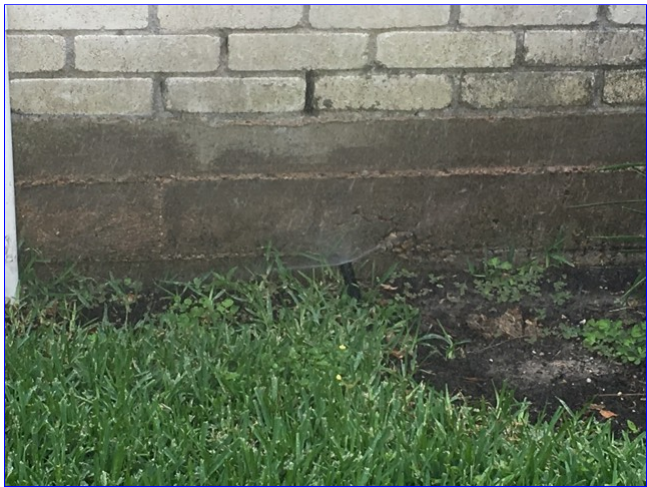
A. Item 4(Picture) Zone three sprinkler head needs to be reset perpendicular to the ground.
