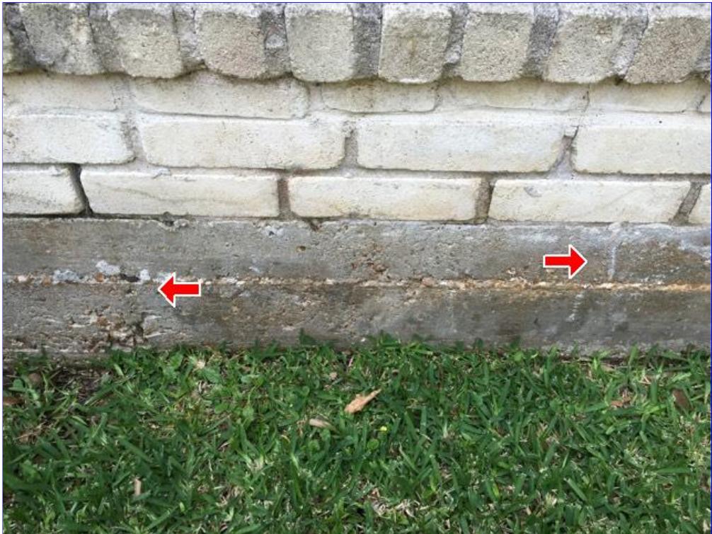
A. Item 3(Picture) Hairline cracks in foundation on right side of home.
