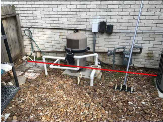
A. Item 1(Picture) Minimum of 4 inches of slab exposure needed at left side of home.
