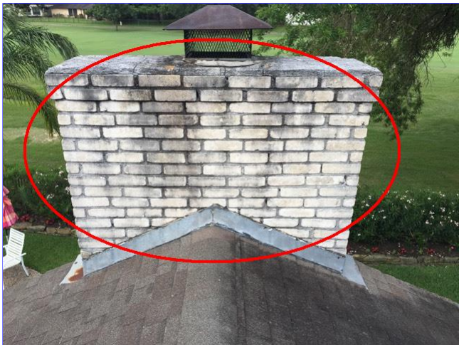
E. Item 13(Picture) Chimney brick has cracks and bee holes in it.
