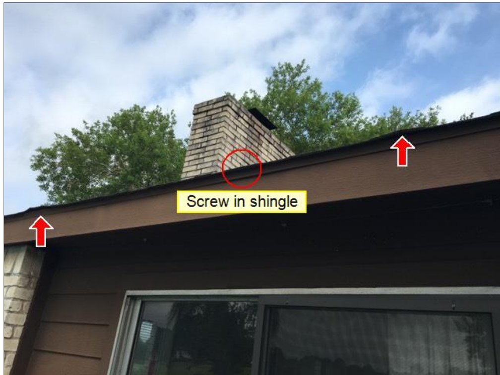
C. Item 1(Picture) Lifted shingles at rear of home. In addition screw in shingle at rear of home.
