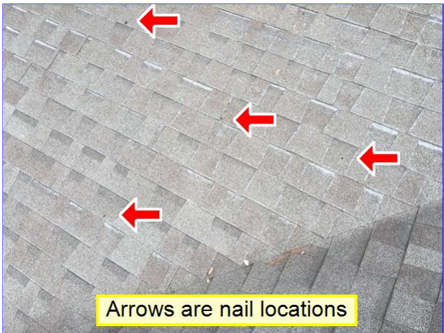
E. Item 11(Picture) Nails hammered through shingles and shingles delaminating had rear slope of home.
