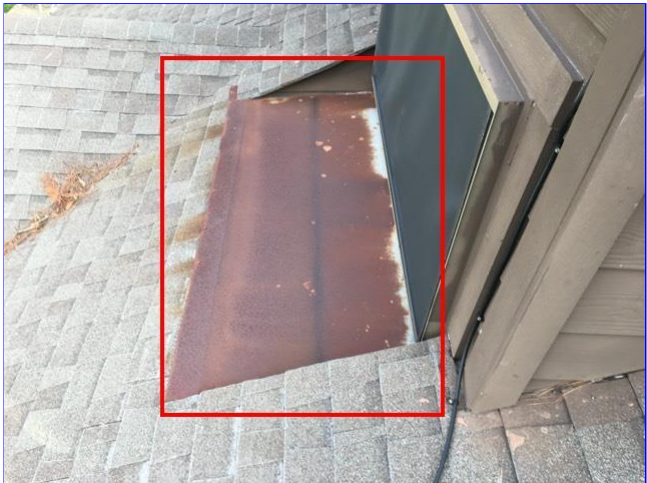
C. Item 17(Picture) Roofing pan needs to be sanded, primed and painted. Nails also need to be sealed at rear of home.
