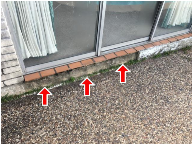
G. Item 1(Picture) Underpinning at rear sliding glass door broken.
