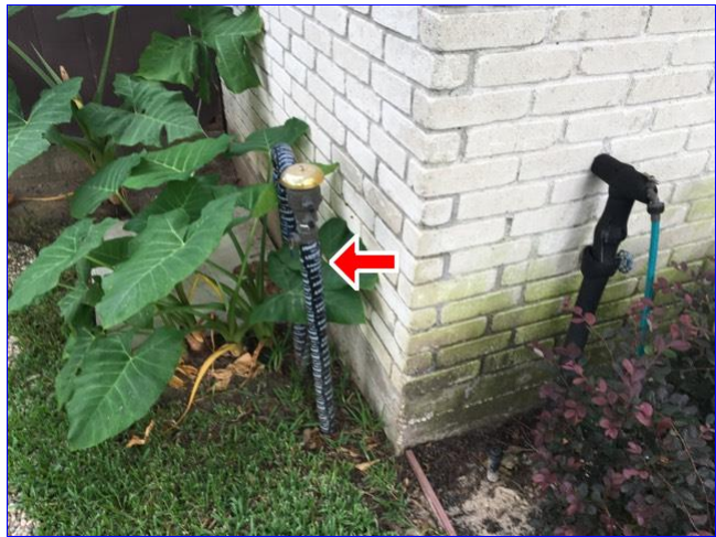
A. Item 2(Picture) Irrigation backflow prevention device should be secured to wall at left side of home.
