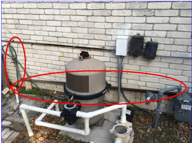
E. Item 1(Picture) Gas line at left side of home needs to be capped. Also signs of rust and corrosion. It is recommended that the gas line be removed and capped.
