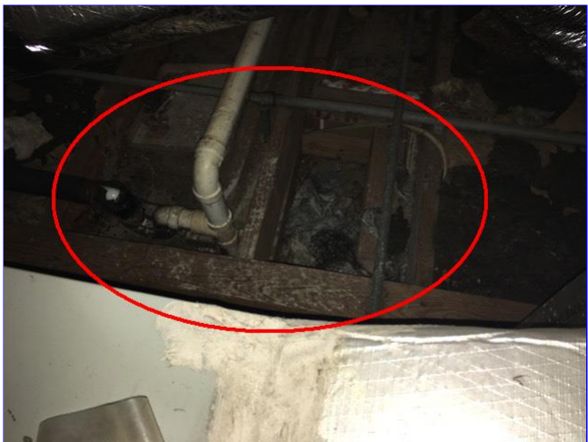
F. Item 3(Picture) Insulation missing above right hall bath. First floor.
