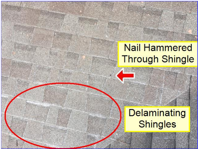
C. Item 22(Picture) Nails hammered through shingles and shingles delaminating at rear slope of home.
