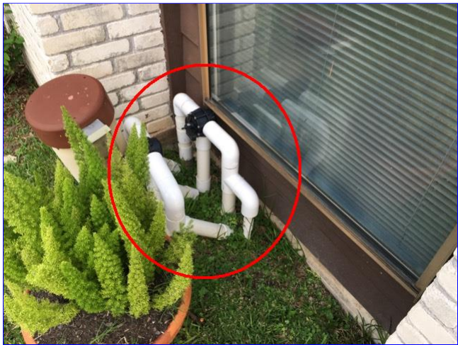
B. Item 4(Picture) It is recommended that PVC pipe being be painted at rear of home
