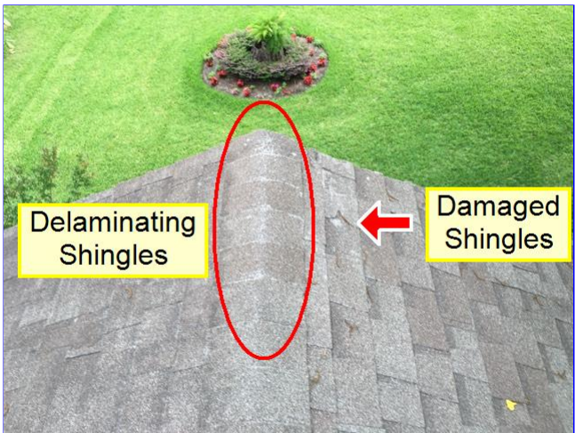
C. Item 5(Picture) Damaged and delaminating shingles at right gable of home.
