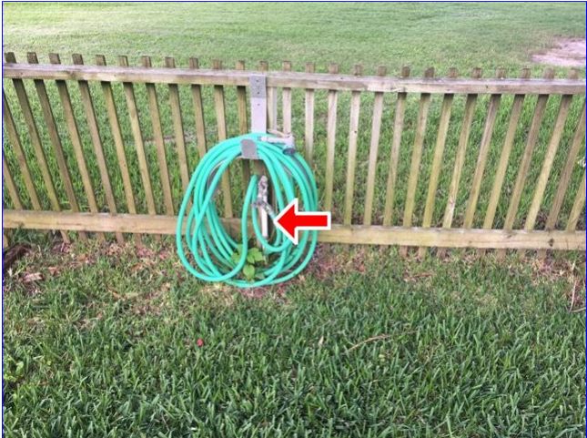
A. Item 3(Picture) Right side hose bib stubs out at rear of backyard. Piping should be insulated.
