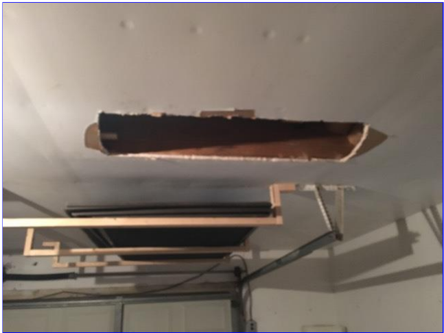
F. Item 1(Picture) Hole in ceiling of garage.
